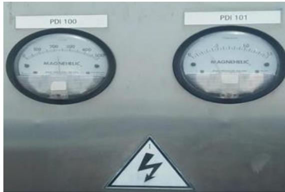
**Gambar 4.** Pressure different indikator PT. ELB
